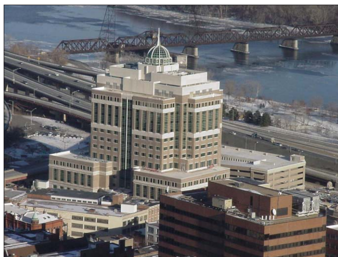
Completed in the spring of 2001, the New York State Department of Environmental Conservation headquarters building in downtown Albany recently achieved a LEED™ Silver rating. Photo courtesy of NYSOGS
